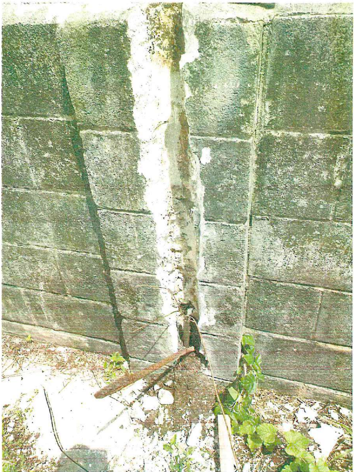
Exhibit A: Impassable conduit at Northwest parking light. Old deteriorated wires could not be removed. Rust debris from old light post visible.
