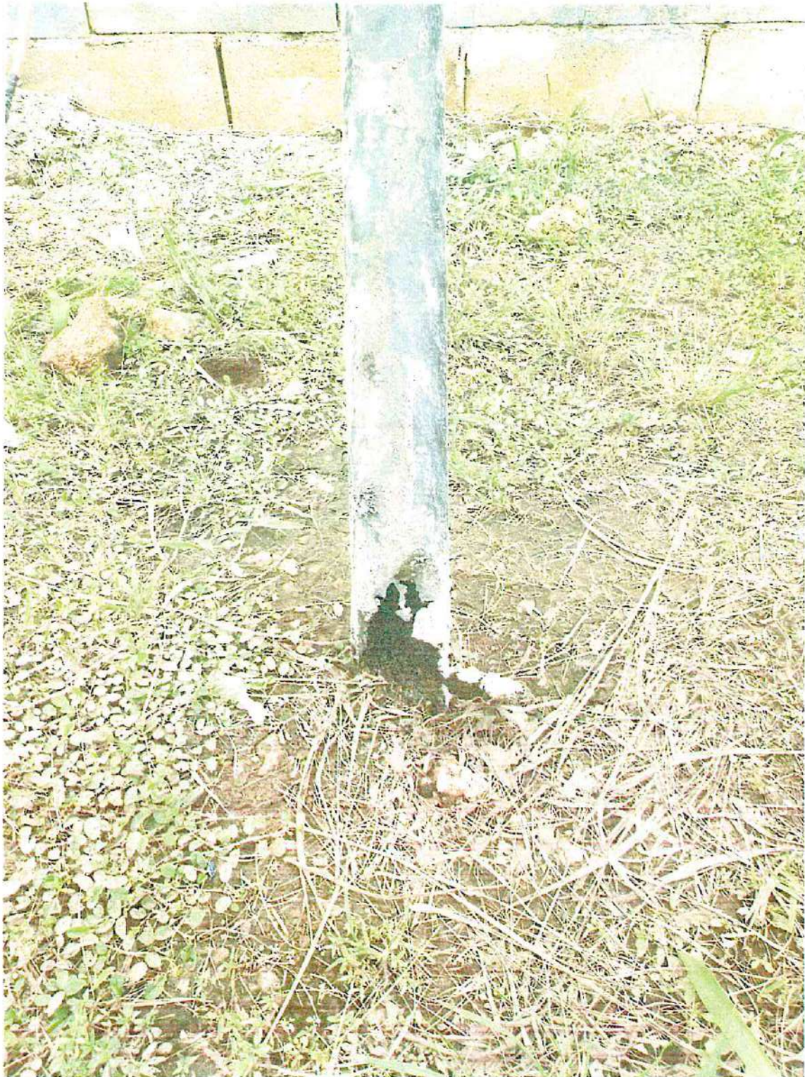
Exhibit A: Condition of light post removed from Southeast parking light. Light gauge steel has rusted entirely causing failure at pedestal.
