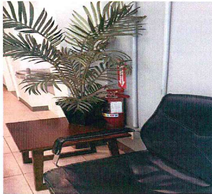
Fire extinguisher hidden behind a table and plant (Lobby).
