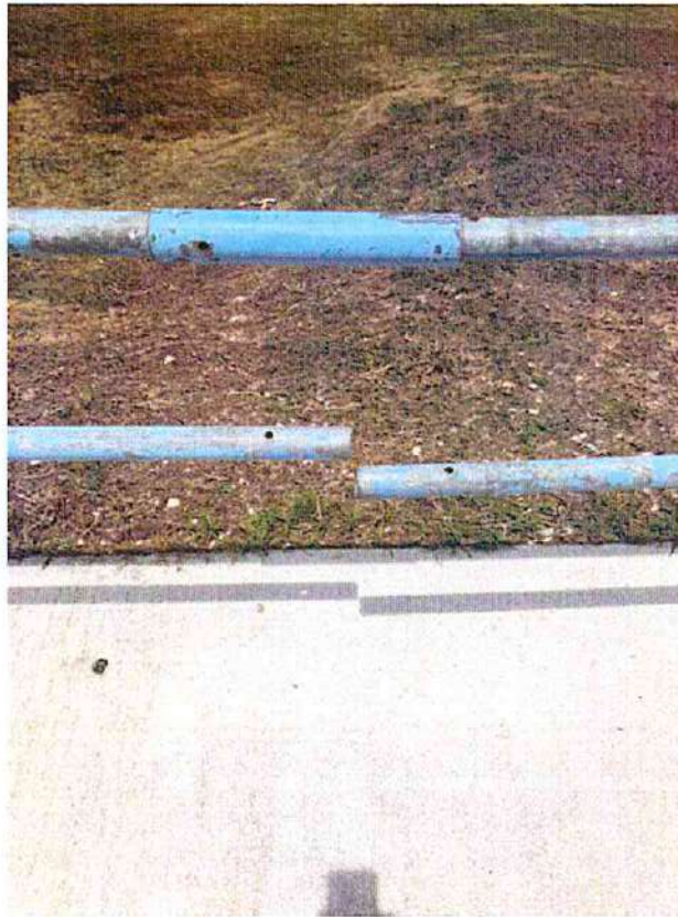
Pipe railings not connected.
