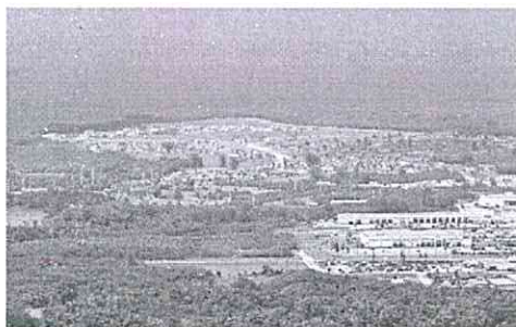
NAVAL BASE GUAM: Naval Base Guam is shown from Santa Rita on Tuesday. Most of the $723 million in proposed military construction projects for Guam in the Trump administration's defense spending proposal for 2021 will be under the Navy. David Castro/The Guam Daily Post
