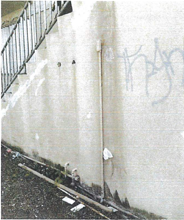
EXPOSED WATER LINE @ BUILDING REAR
