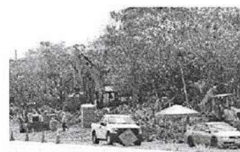
ROADWORK: The Route 3 road-widening project in advance of the military buildup began in April 2018. Legislation introduced recently by Del. Michael San Nicolas proposes to give preference to Native Chamorro contractors for military and other federal projects.
